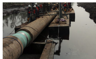
Pipeline reinforced mesh for river bottom gas & oil pipeline transfer
