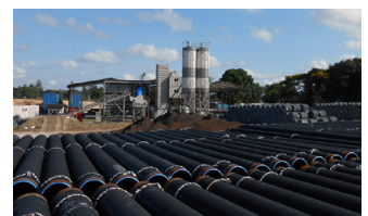
Pipeline reinforced mesh for everglades gas pipeline transfer
