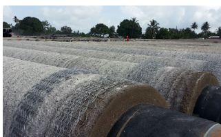
Pipeline reinforced mesh for subsea gas pipeline transfer
